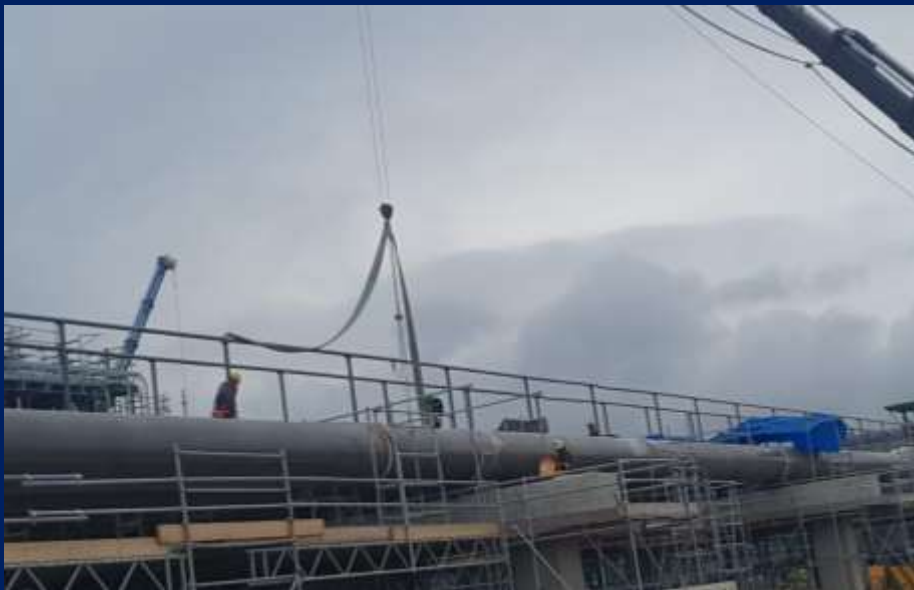
TPOTC- Schlumberger- Sakarya Gas Project Slag Catcher installation
