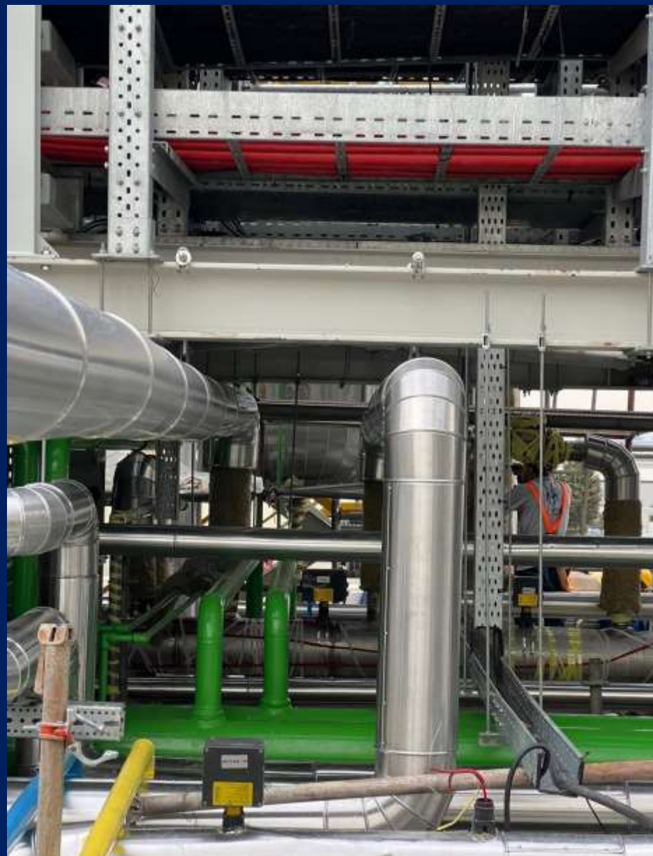
KOCAELI – TATNEFT – TN Maleik Petrokimya- Maleic Anhydride Plant Project Painting and Insulation Works
