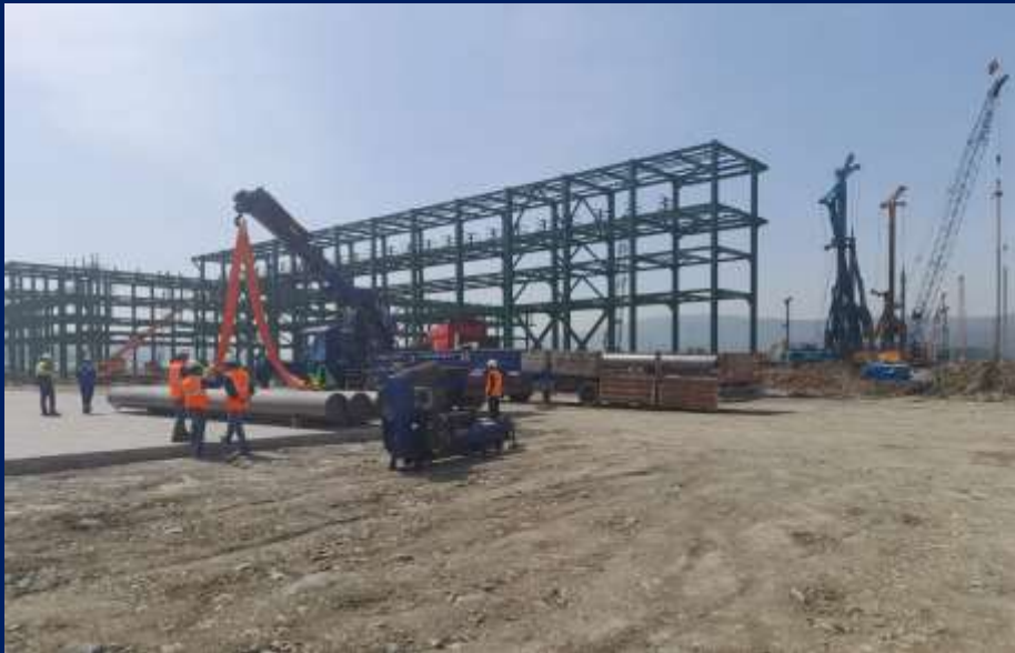
TPOTC- Schlumberger- Sakarya Gas Pipe Erection
