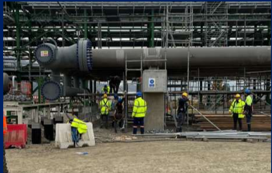
TPOTC- Schlumberger- Sakarya Gas Project Slag Catcher installation
