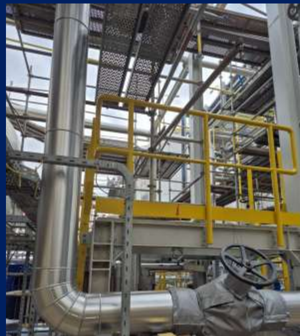
KOCAELİ – TATNEFT – TN Maleik Petrokimya- Maleic Anhydride Plant Project Painting and Insulation Works
